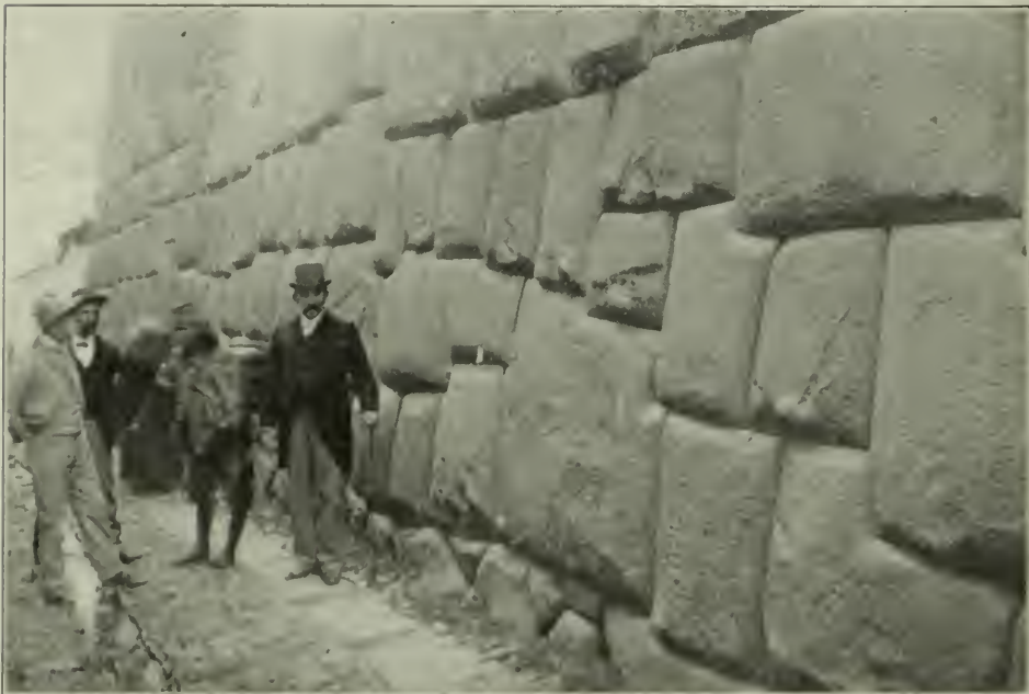
ANCIENT INCA FOUNDATION WALL IN CUZCO, PERU. THOUGH LARGE AND IRREGULAR IN SHAPE THE STONES ARE FITTED TOGETHER SO PERFECTLY A KNIFE-BLADE CANNOT BE INSERTED BETWEEN THEM.
